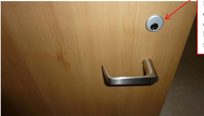
Rotate the mortise cylinder clockwise until it reaches the desired depth and with the key opening oriented in the six o'clock position.
