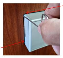
With the door latched, and with the pushbar/pushpad fully extended, Insert supplied Release Tool between the pocket cutout and top corner of the latch-side end cap.
