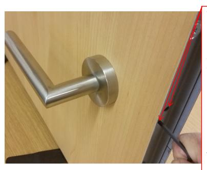
There are two openings in the lock mounting plate in line with the horizontal handle location. Only tighten the setscrew adjacent to the handle being installed.
