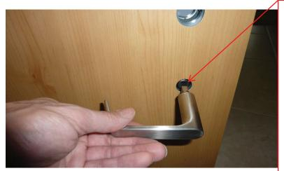
Trip the latch trigger at the top of the door to extend the top latch.
