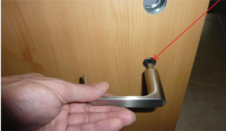
Trip the latch trigger at the top of the door to extend the top latch.
