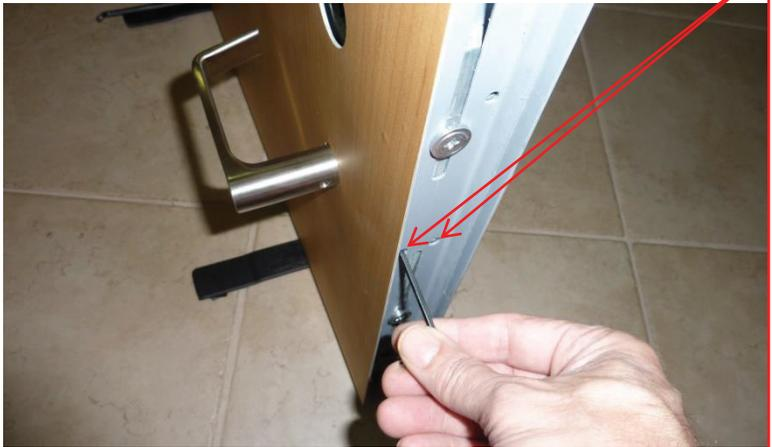
There are two openings in the lock mounting plate in line with the horizontal handle location. Only tighten the setscrew adjacent to the handle being installed.
