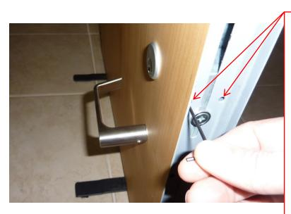
There are two openings in the lock mounting plate in line with the horizontal cylinder location. Only tighten the setscrew adjacent to the cylinder being installed.
