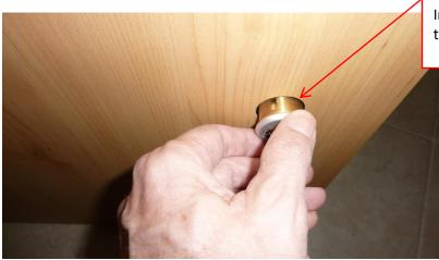
Insert the cylinder into the lock case opening.
