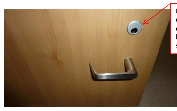
Rotate the mortise cylinder clockwise until it reaches the desired depth and with the key opening oriented in the six o'clock position.
