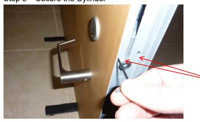
There are two openings in the lock mounting plate in line with the horizontal cylinder location. Only tighten the setscrew adjacent to the cylinder being installed.
