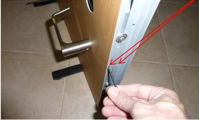
There are two openings in the lock mounting plate in line with the horizontal handle location. Only tighten the setscrew adjacent to the handle being installed.
