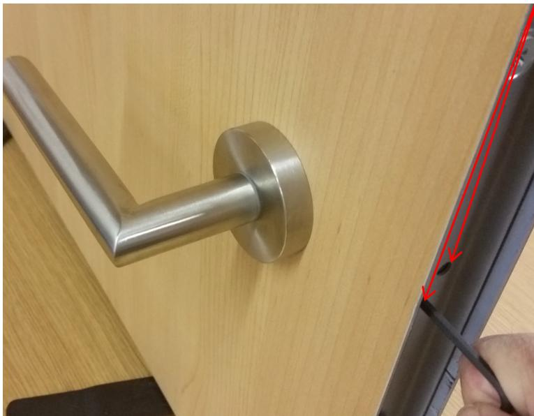
There are two openings in the lock mounting plate in line with the horizontal handle location. Only tighten the setscrew adjacent to the handle being installed.
