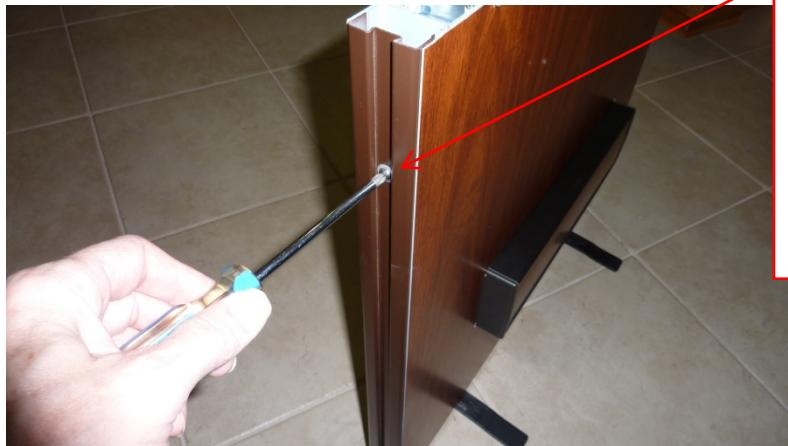
Remove the door edge by loosening all screws along the vertical edge. The screw arrangement varies depending on the door edge configuration.
