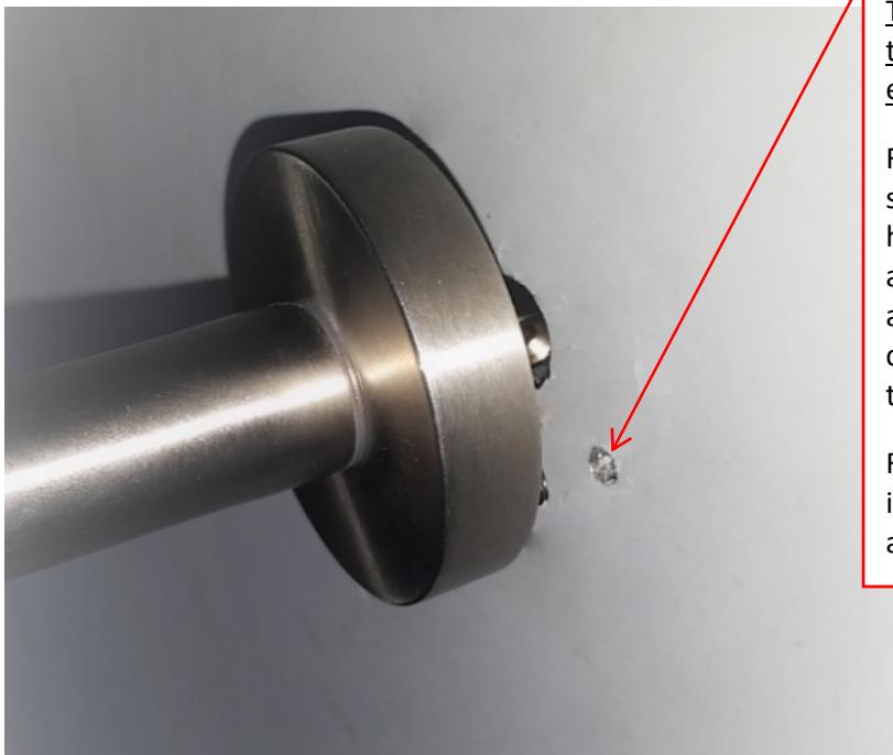
Trip the latch trigger at the top of the door to extend the top latch.
